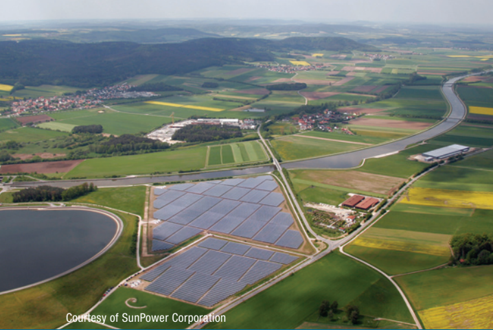
Courtesy of SunPower Corporation
