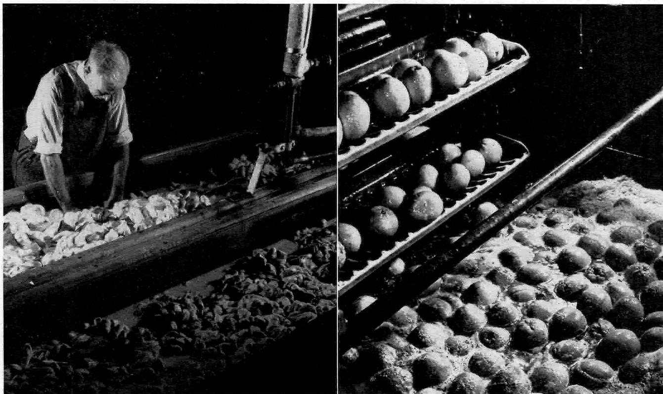
FIG. 5. AT LEFT: Soap has a role in many industrial processes. Here raw silk for parachutes and shroud lines gets a "soaking" bath as an important step in its processing. FIG. 6. AT RIGHT: First step in the packing house in preparing oranges for market is the soap-and-water bath. On the left, a carrier removes oranges from the suds and takes them up to be rinsed with warm and cold showers, then dried by brushes and warm air currents.
