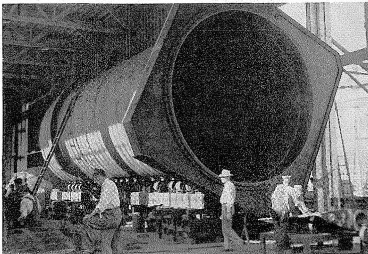
Construction of heavy, specialized pressure vessel at Lacy's.
