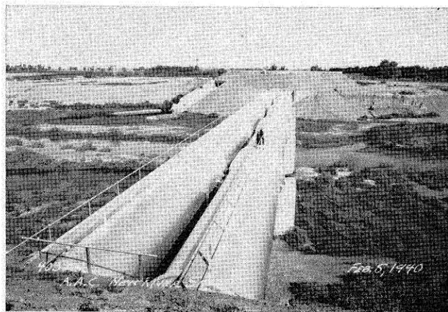
Plate 7. A.A.C. New River Siphon. The pipes are 15' 6" in diameter, and canal capacity at this point is 2600 second feet.
