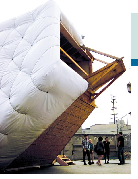
The full-sized mock-up of the SCI-Arc/Caltech Solar Decathlon house is partially covered in a soft, insulated "skin" of architectural vinyl.
