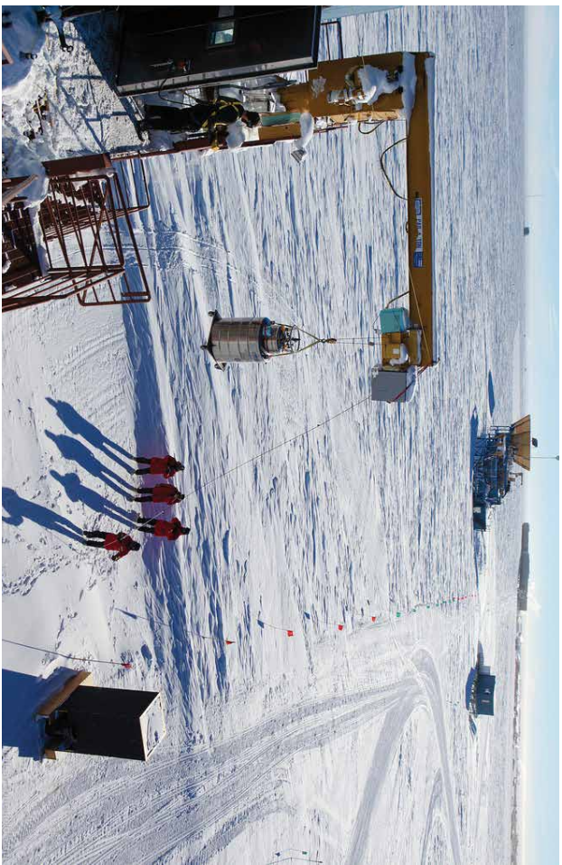
BICEP2 team members lift a liquid helium cryostat to the second floor of the Dark Sector Laboratory to chill the telescope to a temperature near absolute zero.
