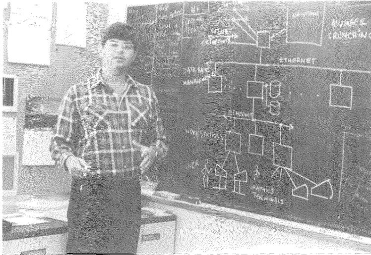
*Paul Dimotakis sketches CADRE's hierarchical architecture, in which a number of work stations, each serving one or more user terminals, are connected via Ethernet to data base management stations, which are joined in turn to the main computer. CADRE will also link up to the campus-wide network already under way, and a system of direct interconnections from the various levels will make CADRE fail-safe.*
