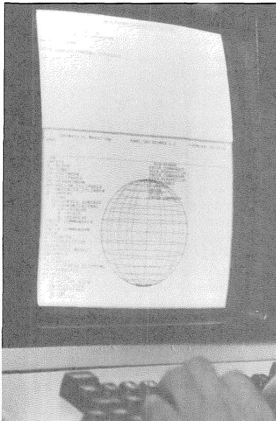
used in the analysis and direct the computer to analyze how it might respond to loads. He could then tell the computer to show him visually how the model would warp in response to a given load.
