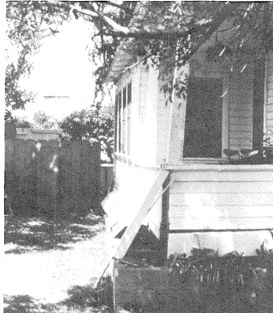
The two pre-1933 residences at the left show the effects of a magnitude 6.5 earthquake — one losing much of its front wall and the other shifting off its foundation.
