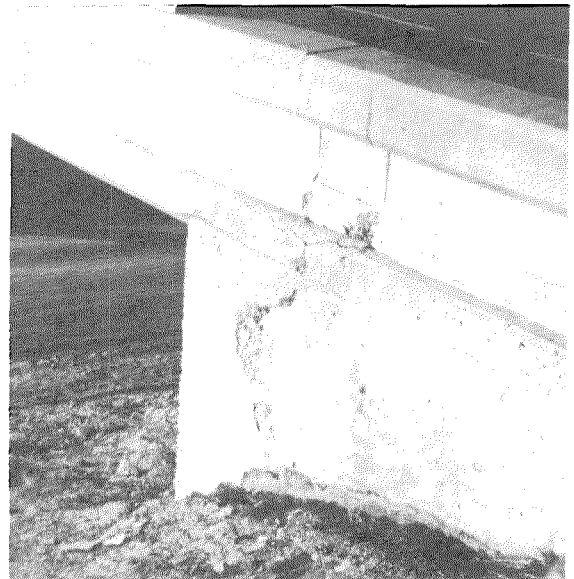
Damage to freeway bridges was fairly minor. An example of spalling is shown at the left and of cracking, above.
