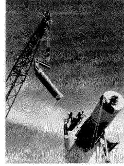
**Right: It took three cranes, manned by a rigging crew of 12, to lift one of the huge dishes onto its pedestal. Securing it in position involved meshing the pedestal gears with the driving gears on the dish, and welding two counterweights of 18 tons each onto the dish before the cranes could release their grip.**
