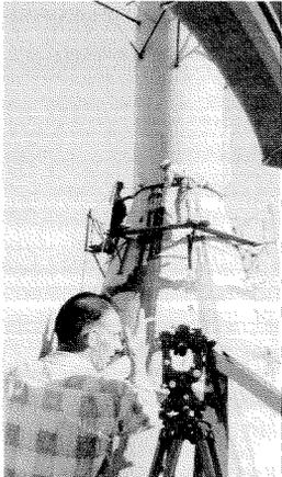
**Bolton, with a theodolite, checks the installation of the top section of the tower for one of the antennas in 1958. Bolton spent a lot of time at OVRO, watching the details of construction and doing some of it himself.**
