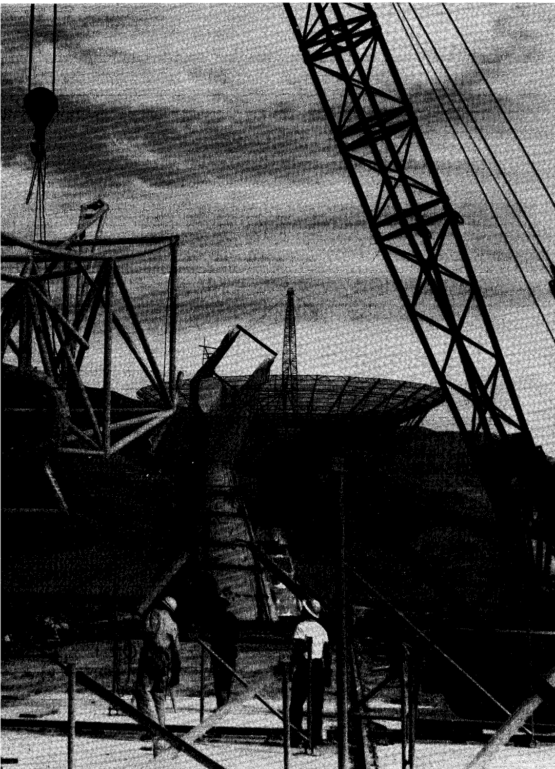
Caltech's first radio observatory begins to take shape in the Owens Valley in the late 1950s. One of the 90-foot antennas of the interferometer stands virtually complete in the background, while the pedestal of the second waits to grasp in its thumb-and-forefinger-like mount the other dish, whose frame is just getting started in the foreground.
