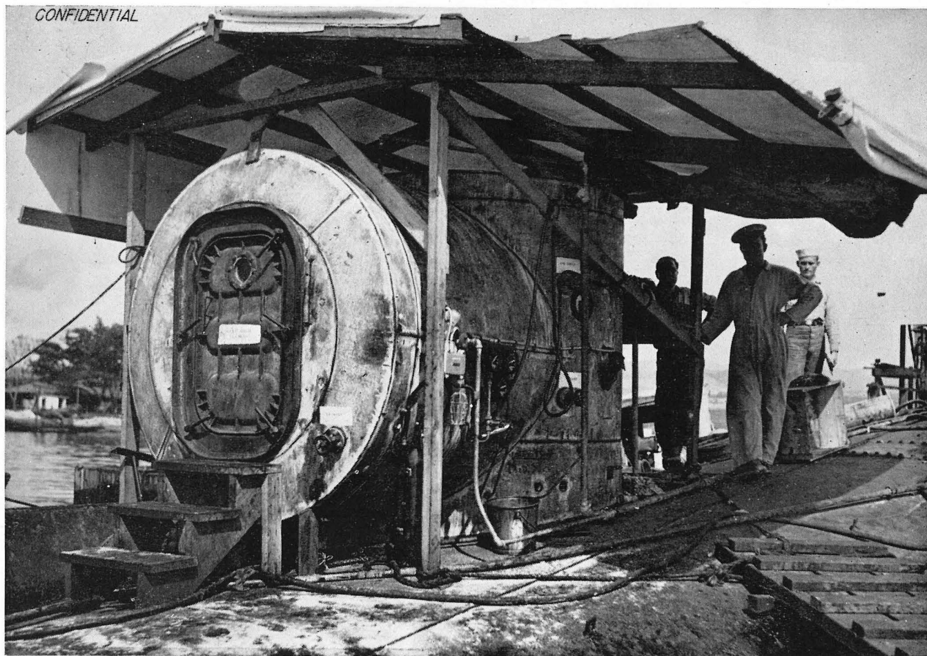
Fig. 12 Airlock for access to and from one section of the main air bubble. The bubble, designed to lighten the ship, was divided into seven sections which extended from stem to stern. It was effective from the bottom to the second deck, originally about 25 ft below the water level. Each air lock while being used was manned by a crew supervised by an officer diver.
