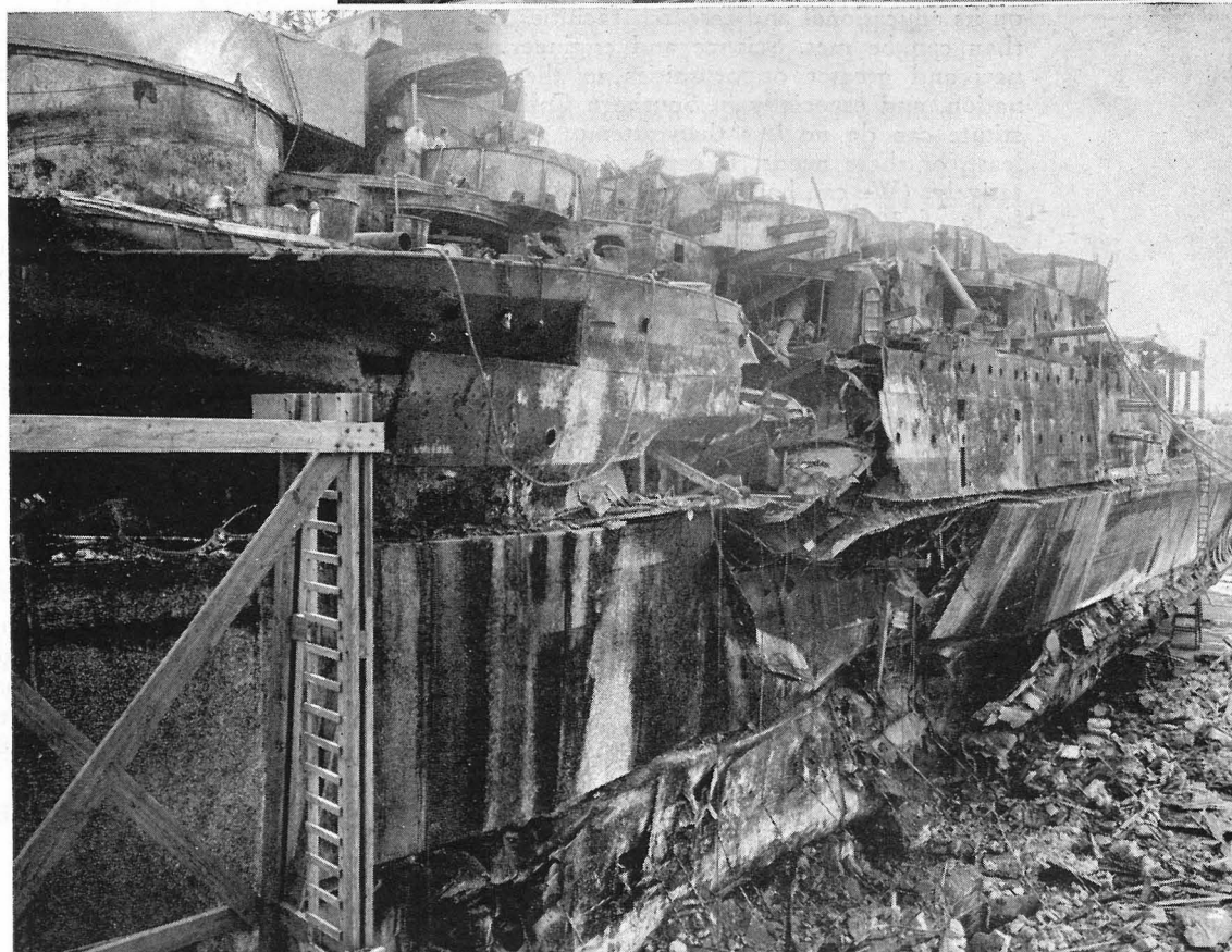
Fig. 24 Port side looking aft after removal of patches. These were removed by cutting the various supporting members. One of the important features in designing the patches was to insure against their premature collapse after the supporting forces of buoyancy and hydraulic pressure were removed when the ship was no longer water borne.
