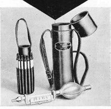
Measures presence of hydrogen sulphide gas in amounts ranging from .0025% to .04%. Any gas present discolors the chemical in the detector to a dark gray—length of discoloration shows degree of concentration. Detector tubes may be marked and kept for several years. Light, convenient to carry, simple to operate.
