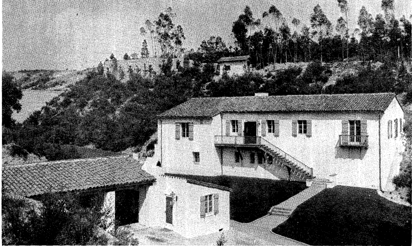
Seismological Laboratory of the California Institute, located in the San Rafael Hills in the western part of Pasadena, where the piers for seismographs are set in firm granite in cuts and tunnels under the building. Photo by Harold A. Parker Studio.
