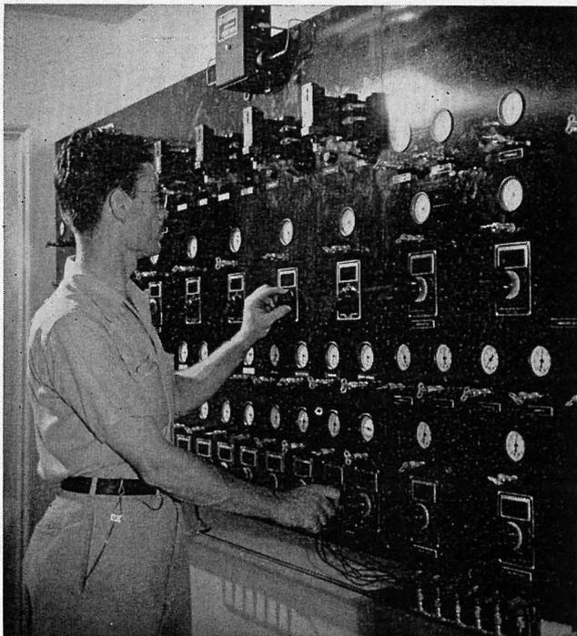
The control room is the brains of the new laboratory. Here, every possible climatic condition can be created.
