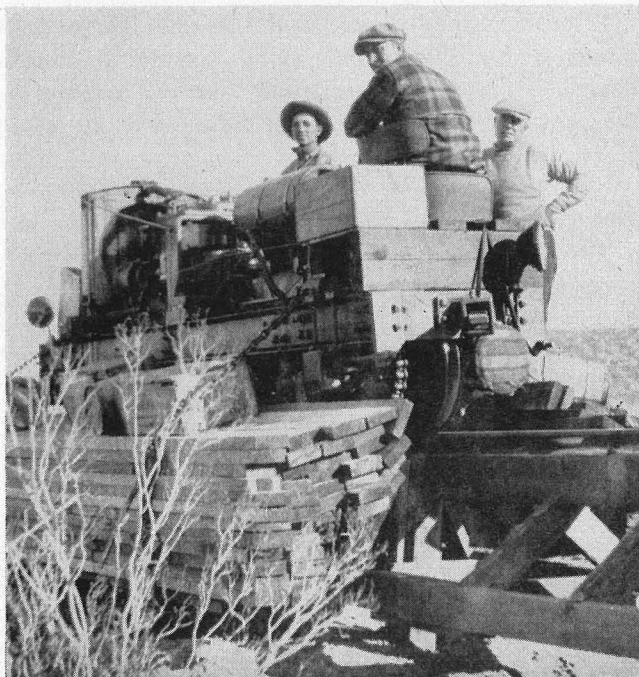
A load of timber, bolts and spikes, during construction days on the line. This was the heaviest locomotive.
