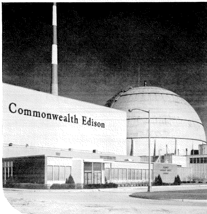
ELECTRIC UTILITY —Built by G.E., the Dresden Station produces commercial electric power from the atom.
