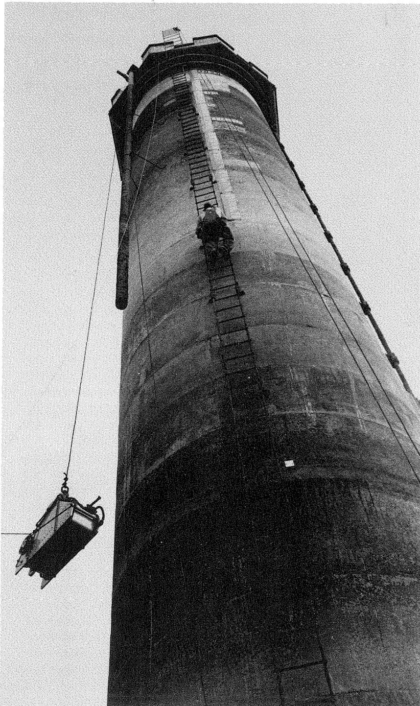
**A Housner-Hudson shaking machine, the first modern earthquake-simulation device, is hoisted to the top of a 110-foot intake tower at the Encino reservoir in the San Fernando Valley for the first field test of the machine in 1961. Although this tower was scheduled for replacement and could be shaken with the energy equivalent to a fairly strong earthquake, a similar machine on Millikan Library jolts that structure only gently for student projects.**
