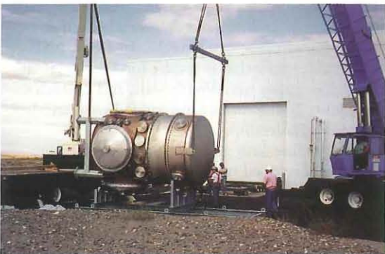
Above: The vacuum tanks arrive at Hanford in August 1997. Right: By February 1998 the vacuum equipment is installed at the point of the L. The center vertical tank houses the beam splitter. At right one of the beam tubes takes off into the desert.
