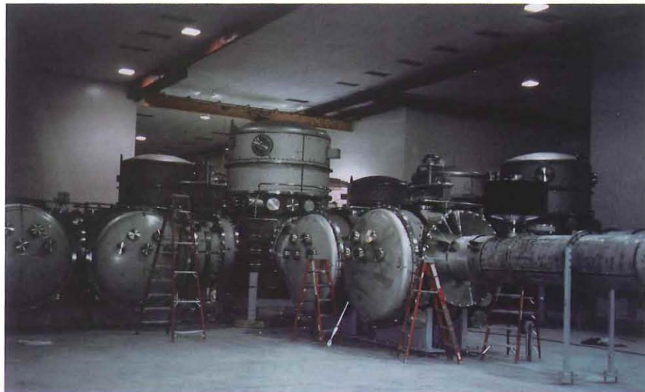
Above: The vacuum tanks arrive at Hanford in August 1997. Right: By February 1998 the vacuum equipment is installed at the point of the L. The center vertical tank houses the beam splitter. At right one of the beam tubes takes off into the desert.
