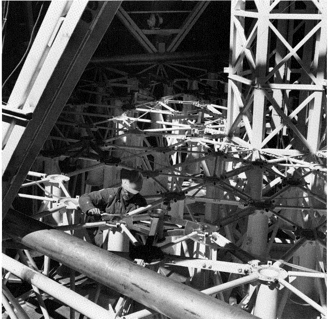
The support structure for Keck I's primary mirror was assembled in Tarragona, Spain.
