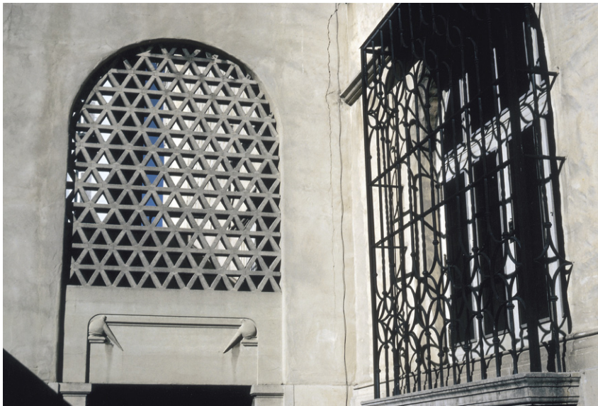
Bridge Annex with two distillation flasks below an arch. The geometrical stone lattice-work filling the arch is similar to mashrabiyya grilles used in Muslim architecture to provide privacy but allow breezes to cool the interior.
