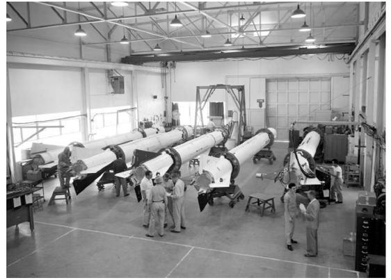
**Corporal missiles being assembled at JPL. This building was later used to build the Mariner and Ranger series of spacecraft.**
