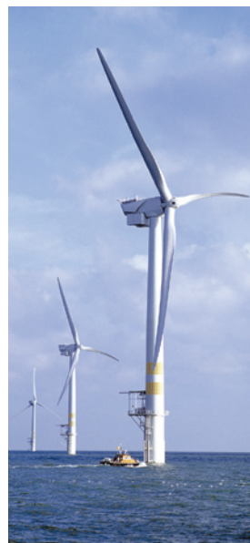
Above, left: Figure 4-14 of the NCEP report shows the parts of the country where solar and wind power is just sitting there for the taking on commercial scales, if people were so inclined to build facilities to capture it. Above, right: General Electric Wind Energy built these 3.6-megawatt wind turbines for a wind farm 10 kilometers off the coast of Arklow, Ireland. The rotors sweep out circles 104 meters in diameter.
