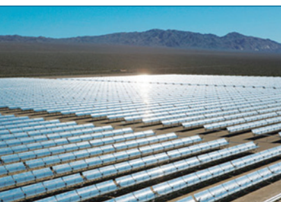
Power production without smokestacks. The Nevada Solar One facility, left, has been running since June 2007. The third-largest facility of its kind in the world at the moment, it puts out 64 megawatts—enough to supply over 14,000 households. The Superphénix fast-breeder reactor, right, in Creys-Malville, Isère, France, was decommissioned in 1997.
