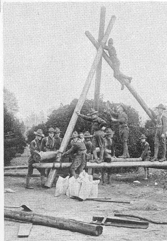
ABOVE — Military engineering trainees get some first-hand experience in derrick erection.
