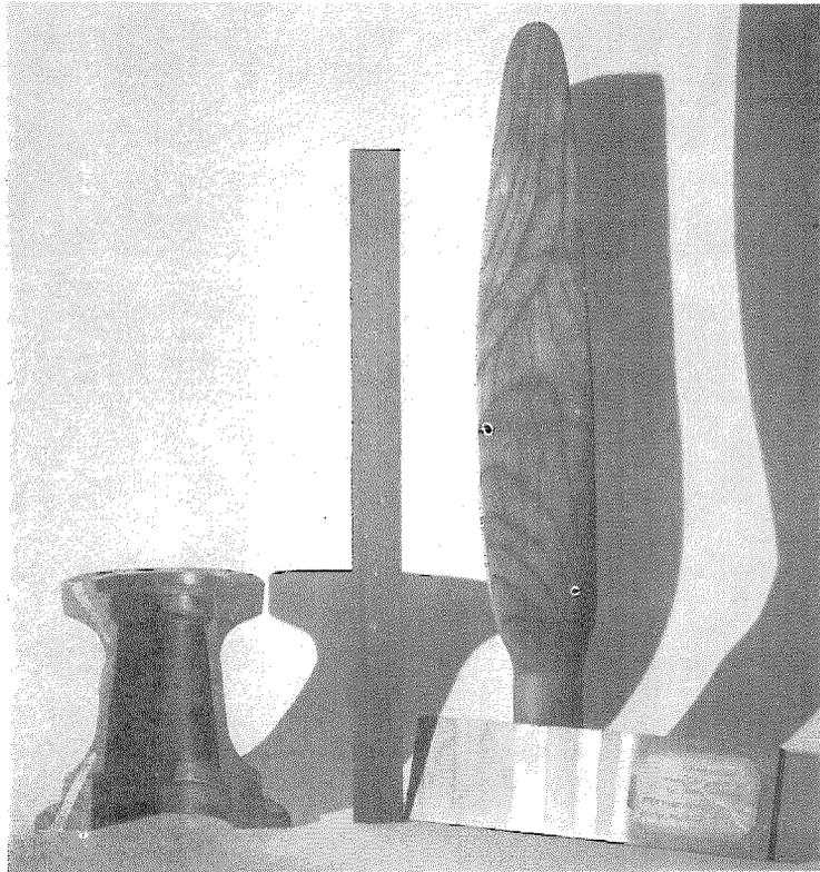
FIG. 4—Left to right, half of an airplane tail wheel molded of compreg; a compreg specimen varying in specific gravity from end to end (1.3 to 0.6); a model airplane propeller molded of compreg; a cut panel of birch compreg sanded and buffed to show that the finish exists throughout the structure.
